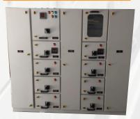
Power Distribution Board (PDB)/ LT panel is an electrical component that is used to distribute electrical power into subsidiary circuit by a circuit breaker and switch fuse unit. It not only ensures efficient distribution of power, but also protects the subsidiary circuits in case of overload and short circuits.
